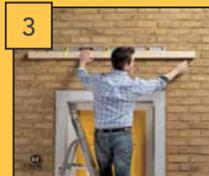
Measure and mark to the wall the back purlin preferred position above door (Fig 3).
