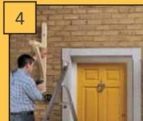
Offer and fix the assembled Gallows Brackets to the pre-marked wall positions and fix using 2 x 12mm Steel Bolts (\*not supplied). Glue the timber cover caps supplied to hide fixings (Fig 4).
