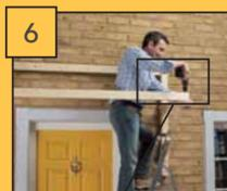
Use a rafter as a guide to establish the exact location of the front purlin to the top of the Gallows Brackets. Fix the front purlin to the Gallows Brackets using the Metal Angle Brackets and 35mmscrews supplied (Fig 6).
