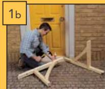
Assemble the Gallows Brackets using exterior grade wood glue (Fig 1a). Knock the 15mm diameter dowels supplied into the pre-machined draw-bored tenons (Fig 1b).
