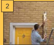
Measure and mark the Gallows Brackets positions on wall to a maximum span of 1600mm (Fig 2).
