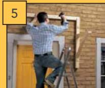
Fix the back purlin to the wall using minimum 2 x 100mm frame fixings or similar (not supplied) (Fig 5).
