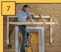
Measure the rafter's positions to the front and back purlins to space out evenly. Fix the rafters to the purlins using the 100mm screws supplied (Fig 7).
