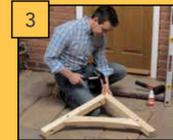
Knock the 15mm diameter dowels supplied into the pre-machined draw-bored tenons (Fig 3).
