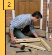
Assemble the Gallows Brackets using exterior grade wood glue (Fig 2).
