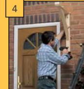
Offer and fix the assembled Gallows Brackets to the pre-marked wall positions and fix using 2 x 12mm Steel Bolts (not supplied). Glue the timber cover caps supplied to hide fixings (Fig 4).
