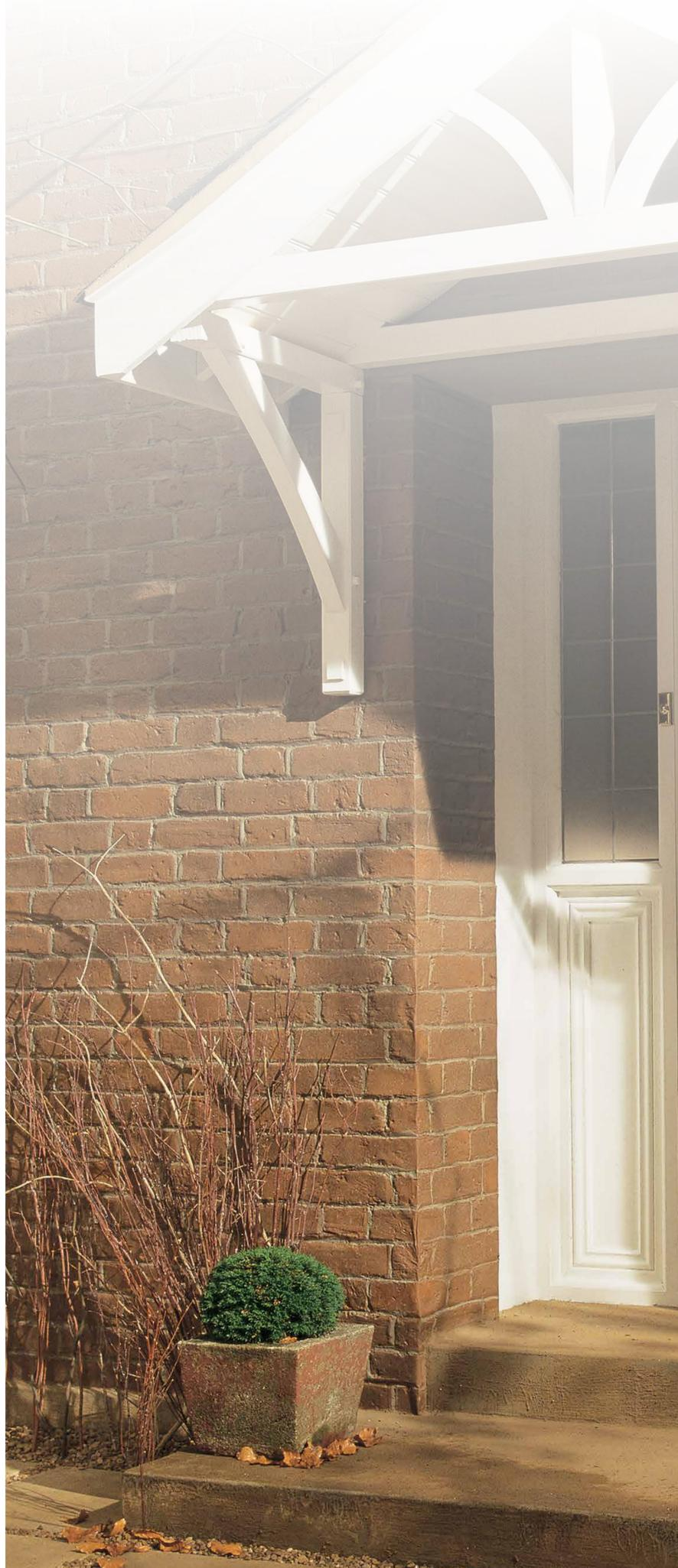
Richard Burbidge Porch Canopies have been structurally tested to hold a maximum weight loading of 50kg/m<sup>2</sup>. Structural calculations are based on fixing to masonry surfaces such as brick, block and stone. If fixing to other surfaces such as timber, we recommend you seek professional guidance/advice via a structural engineer.
